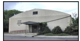
New boiler for Luseland & Community Homecoming Hall $15,000.00
